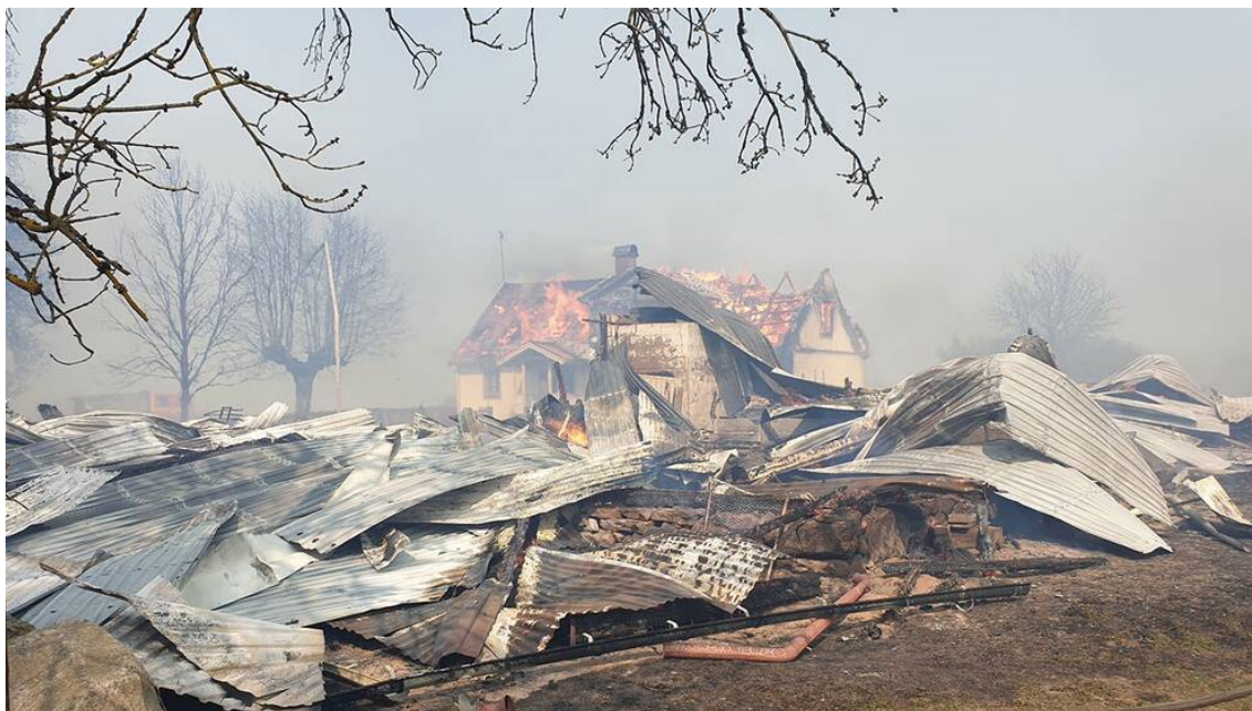
Figure 13. Collapsed stable (foreground) and burning dwelling (background) on the horse farm, 2019. Photo: Mikael Nilsson.
