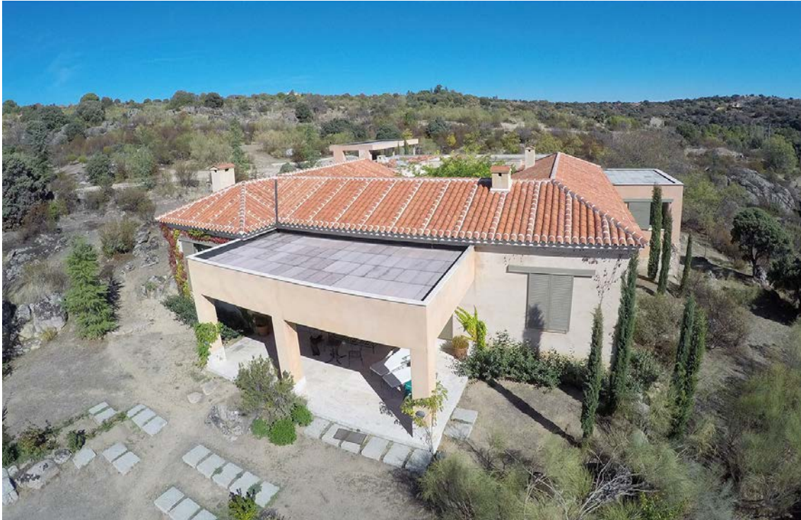
Figure 41. A view of the South-East side with the porche and the surrounding vegetation. Note that some of the ornamental species are touching the façade. Also note the tree inside the patio
