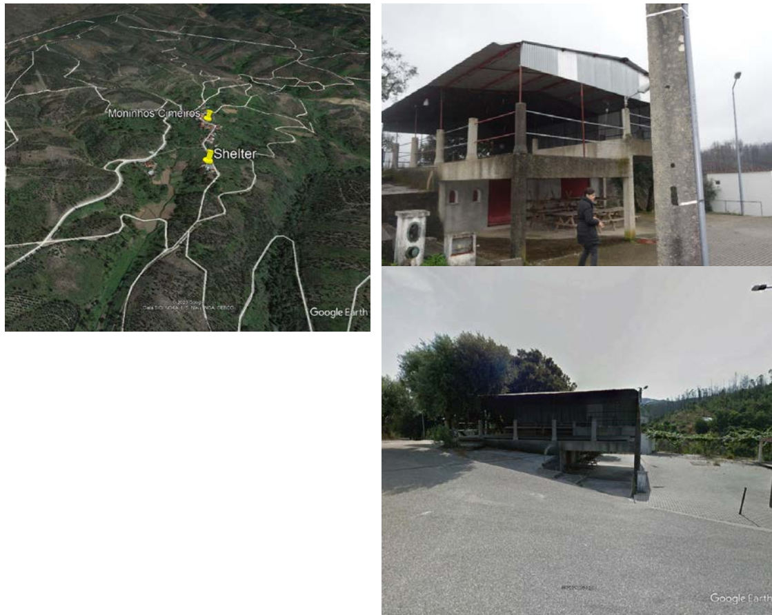
Figure 51. a) Overview of the location of the shelter with respect to the Moninhos Cimeiros village; b) Current state of the structure.
