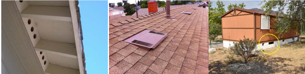
Photo source: D. Caballero; https://ucanr.edu/sites/fire/Prepare/Building/Vents/
